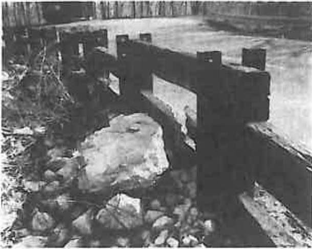
Fig. 2: Brocken tie within a rail and tie wall near Kirchheim/Teck FRG.
