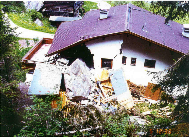
Fig. 1: House at See, Austria, completely destroyed by a 30 m 3 monolithic rockfall in 1995.
