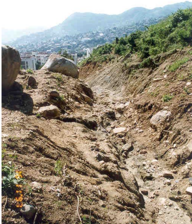
Figure 2. Gully below the crest of the Sierra Madre del Sur after Pauline; banks and bed have been deeply eroded; sandy silts with a high amount of pebbles are exposed.
