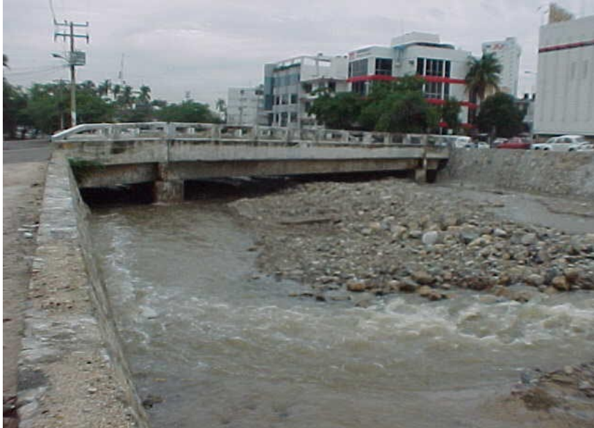
Figure 10. Andrés de Urdaneta Bridge over Arroyo Palma Sola Camarón, before rehabilitation.
