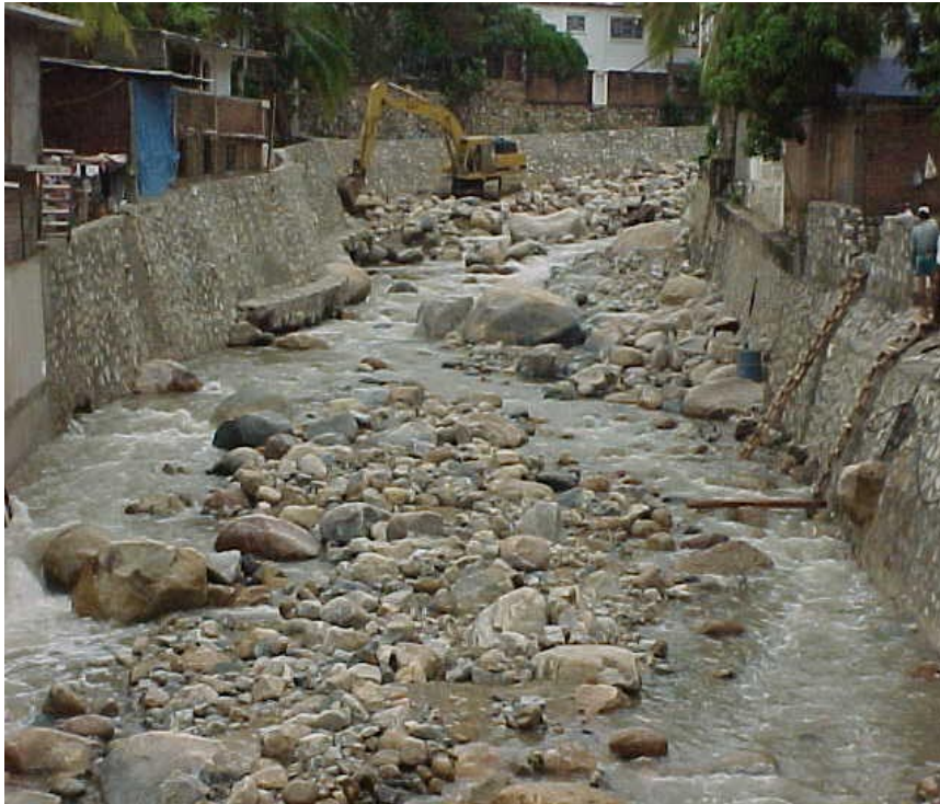
Figure 11. Drainage channel Arroyo Palma Sola Camarón during repair of walls.
