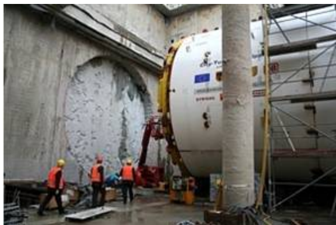
Fig. 6: Preparing of tunneling machine
