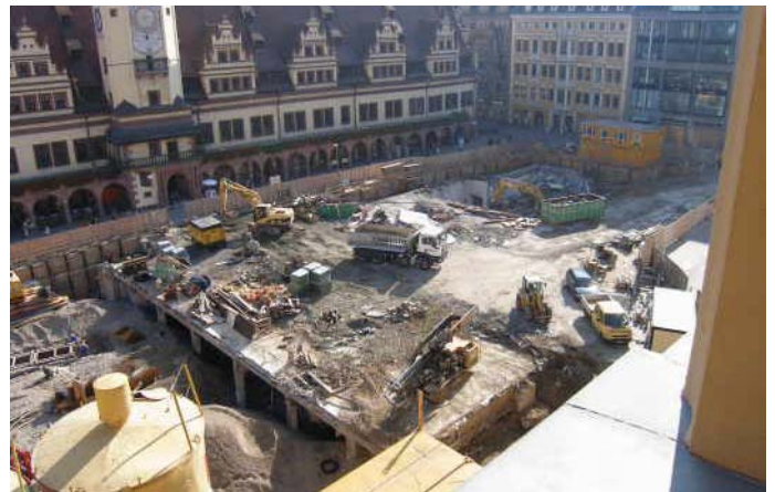
Fig. 5. Construction site of station Markt
