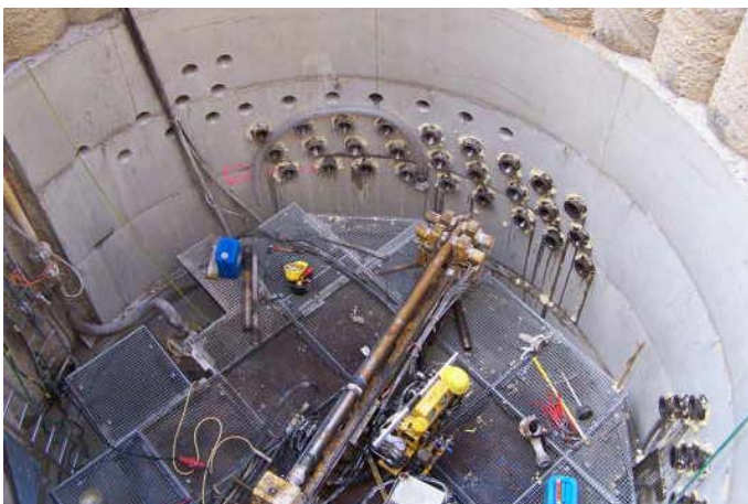
Fig. 7: Shaft and horizontal drillings for the CGV
